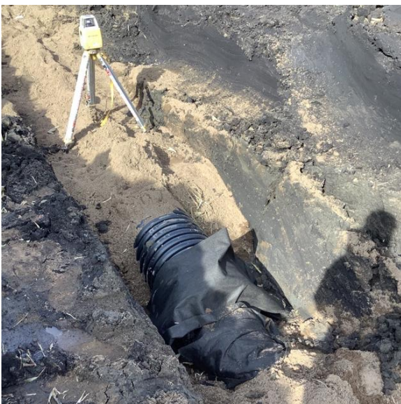
Figure 2: Le Sueur County Ditch 61, November 5, 2021
