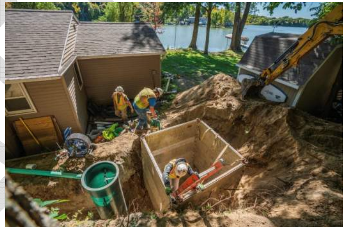
West Jefferson Sewer Construction
