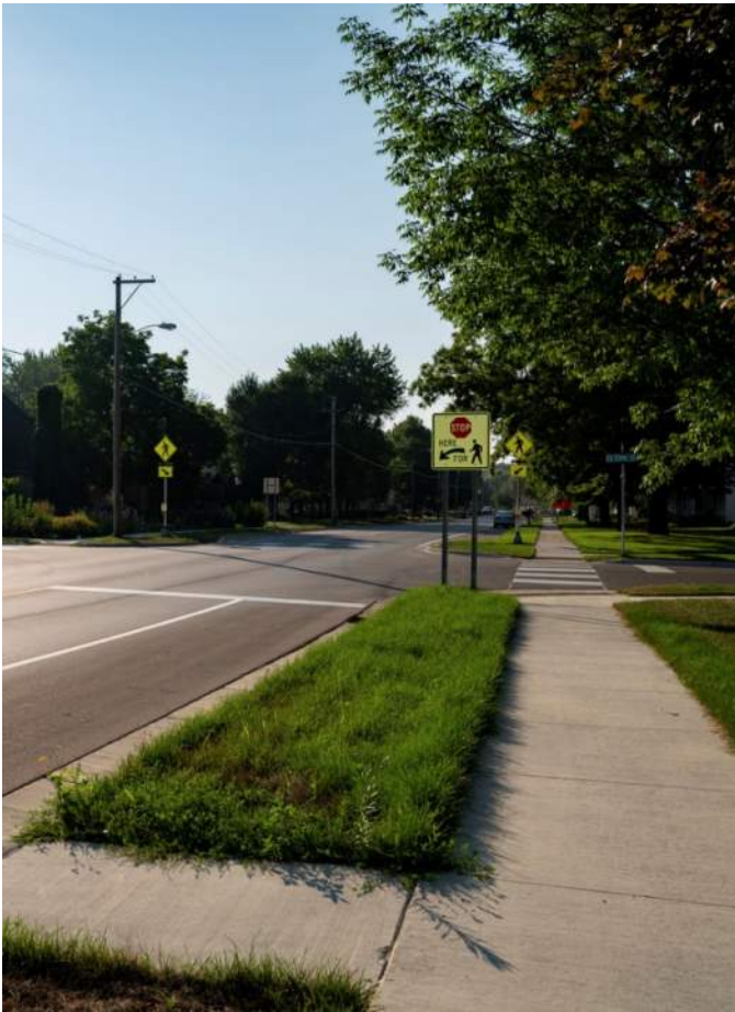
T.A.P. Sidewalk Project
