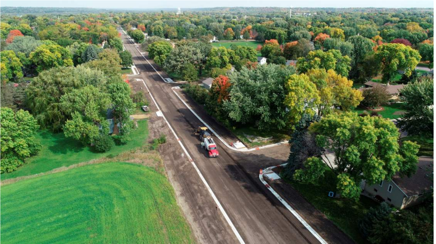
Trunk Highway 112 Turnback Construction
