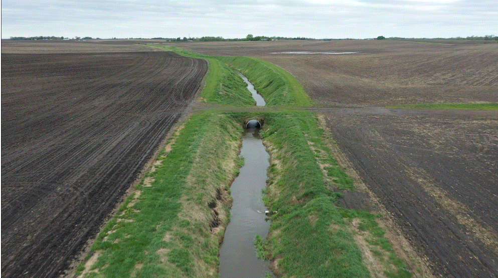
Figure 5: Le Sueur County Ditch 58, May 8, 2020
