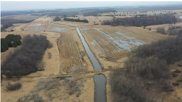
Figure 4: Le Sueur County Ditch 23, March 26, 2021
