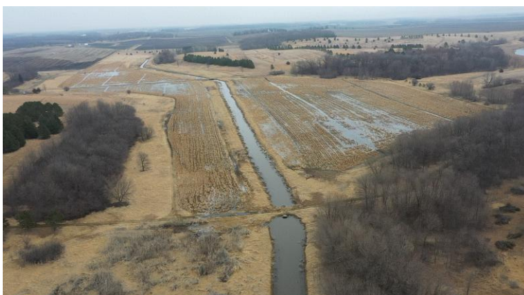
Figure 4: Le Sueur County Ditch 23, March 26, 2021
