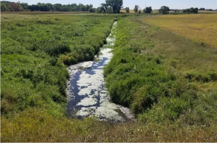
Figure 3: Blue Earth - Le Sueur County Judicial Ditch 15, September 18, 2020
