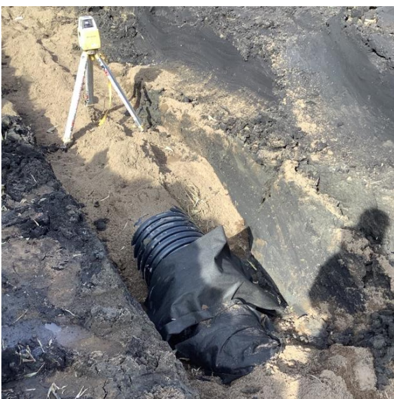
Figure 2: Le Sueur County Ditch 61, November 5, 2021
