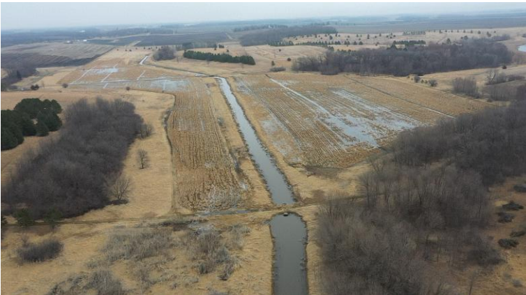
Figure 4: Le Sueur County Ditch 23, March 26, 2021
